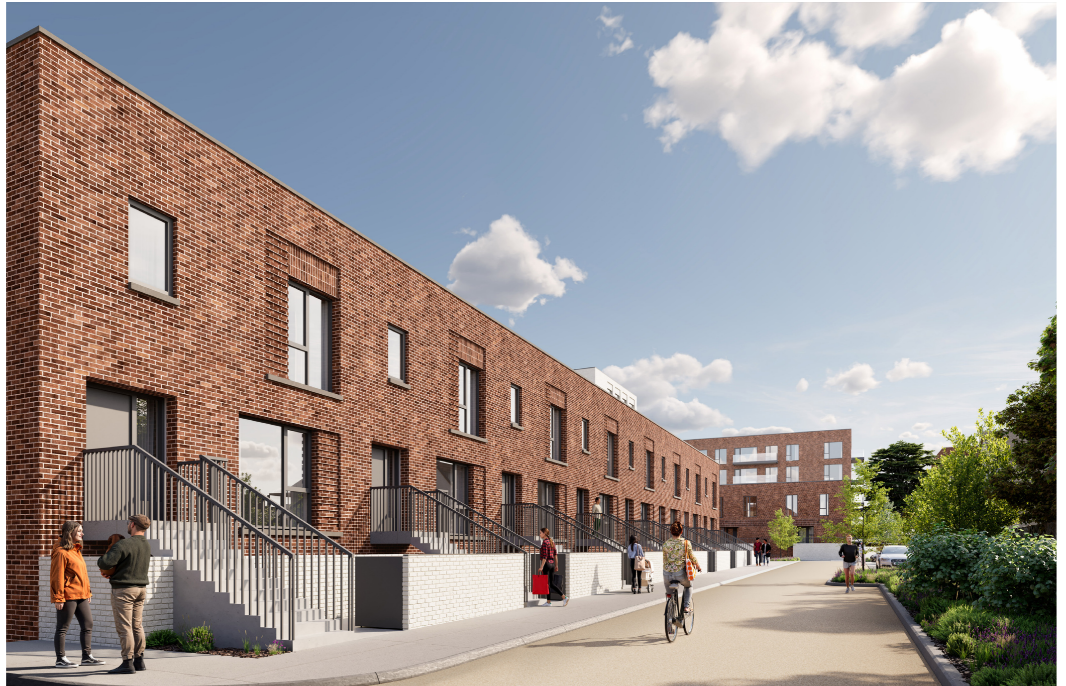
Revised duplex facade, with additional brickwork detailing to the large upper floor windows, with a recessed side and head panel, and stacked soldier courses within the recess.
