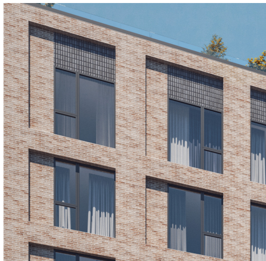
Precedent Image: Brickwork detailing, with recessed panel beside windows, and recessed soldier banding in contrasting brickwork
