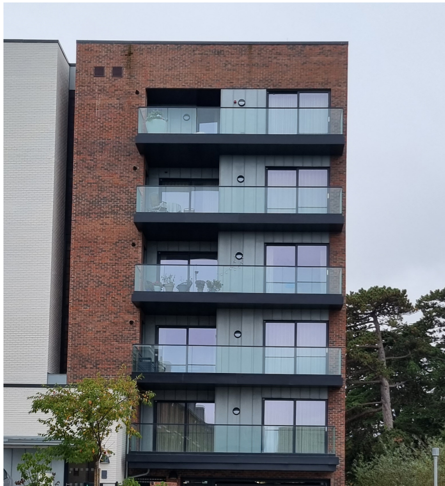
Photo of Block A facade, Phase 1 Knockrabo, with red brick, white brick, zinc cladding, aluminium trim to glass balconies
