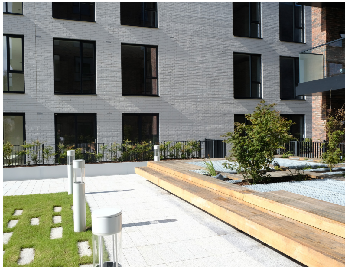
Hard and soft landscaping to communal courtyard
