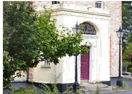
Existing Front Entrance Lobby, Cedar Mount
