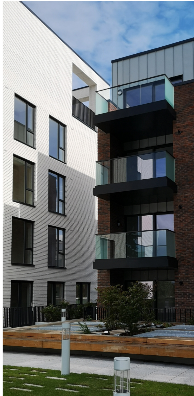
Blocks A & B, with white and red brick, and zinc cladding
