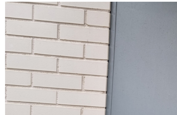
Junction of white brick with zinc cladding
