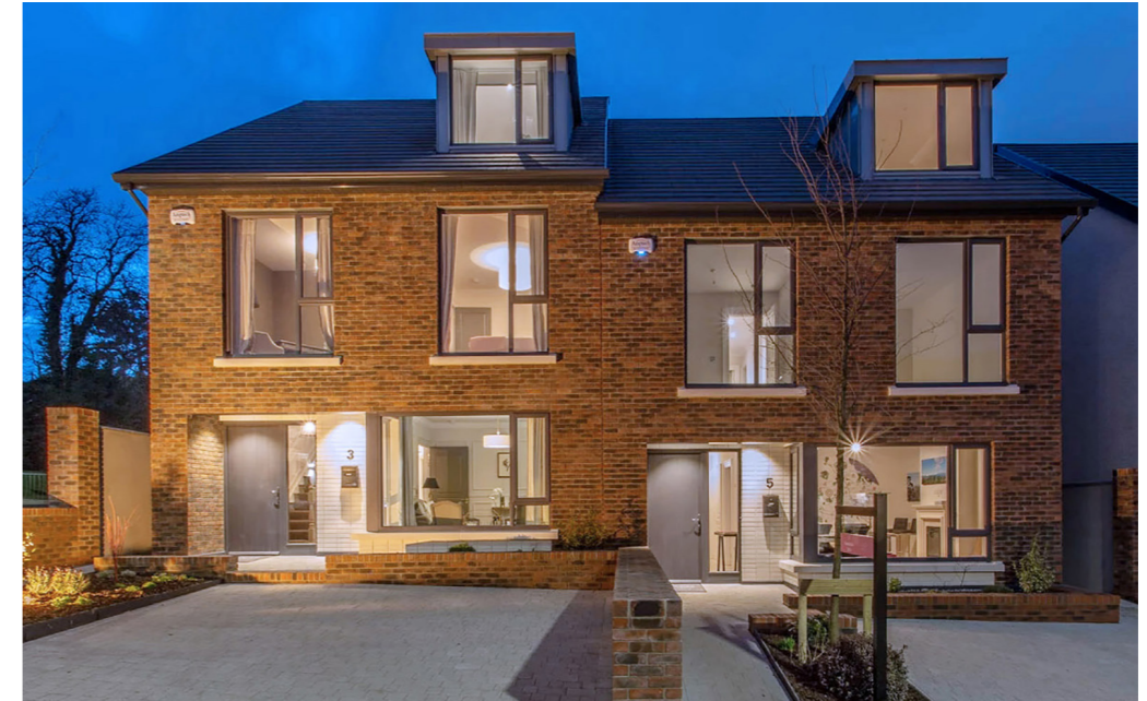
Completed houses in Knockrabo Phase 1, where the changes in level, recessed entrance with contrasting brick & the zinc dormer windows provide variety within the streetscape
